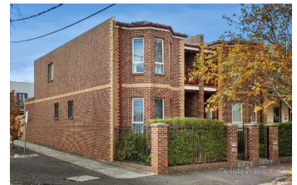
Recent Sale 18a Middle Street, Ascot Vale Sold: June 2017 - $1,200,000 Accommodation: 3 Bed / 2 Bath / 2 Car
